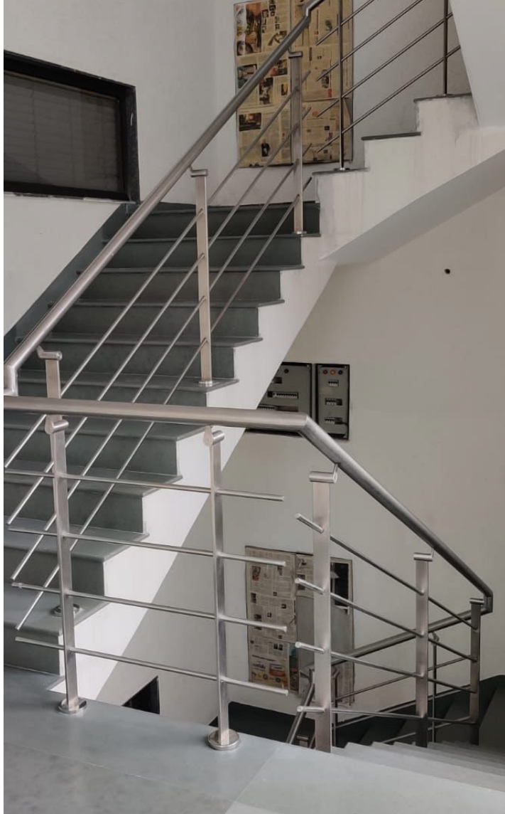
Top-40/50mm SS Round Pipe Square tube Upright-40mm Square/round tube Midrail-16mm dia pipe(3/4nos) Fittings-Midrail 19mm stud holder Grade-304AISI Finish-Matte/Glossy
